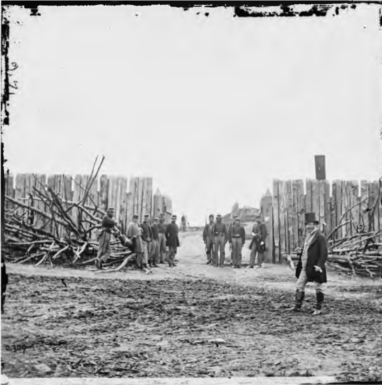
Image of the rear entrance to Fort Corcoran
